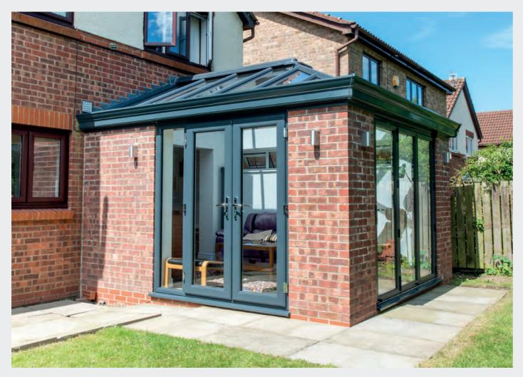
Subtle design differences distinguish Orangeries from the modern day Conservatory, such as a more substantial brick built frame, with conventional walls, fewer windows and a traditional solid roof, usually with skylights.
