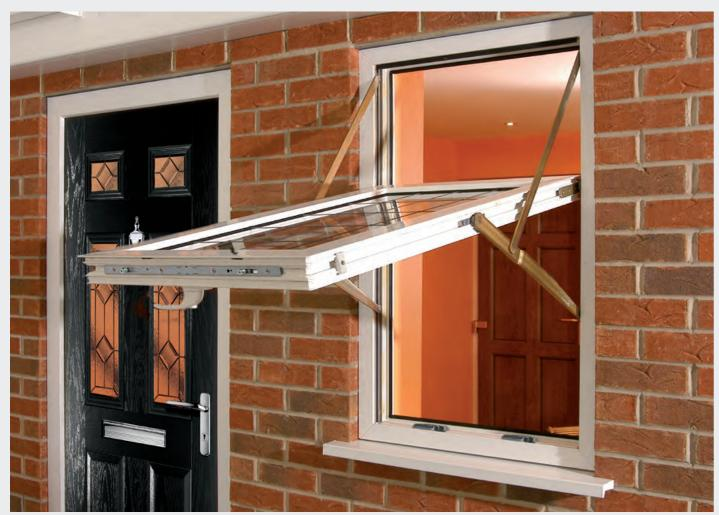
The benefits of Fully Reversible Windows are obvious where window cleaning isn't as simple or accessible as in a ground or first floor home. All moving parts of the windows remain outside, making it less likely that window cleaning liquids will drip into your home.
